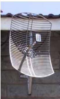
Small parabolic antennas are used on the building(s) at the remote sites to receive and transmit traffic. In this way organisations can minimise the number of connections that they have to external telcos and ISP's enabling them to improve security and manage costs.
